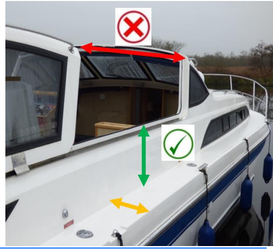
Fig 12. In this example the gap between the cabin roof handrails is greater than 1.5m and is therefore not compliant. However, even though the side deck is less than 300mm wide, the top of the coaming (which the hire operator has designated as a handhold) is greater than 350mm above the side deck, which is compliant.
