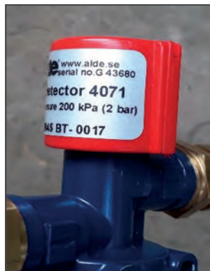
Figure 2. '4071' should be clearly visible on a label on the red test button.
