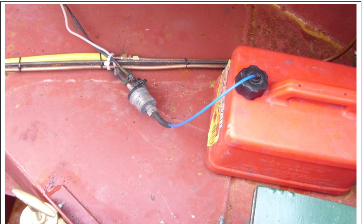
Fig 2. Spare fuel containers, such as the one shown in this photograph, cannot be accepted as diesel appliance tanks of suitable proprietary manufacture as they will not have been manufactured for such use or sold by the appliance manufacture for such use.
