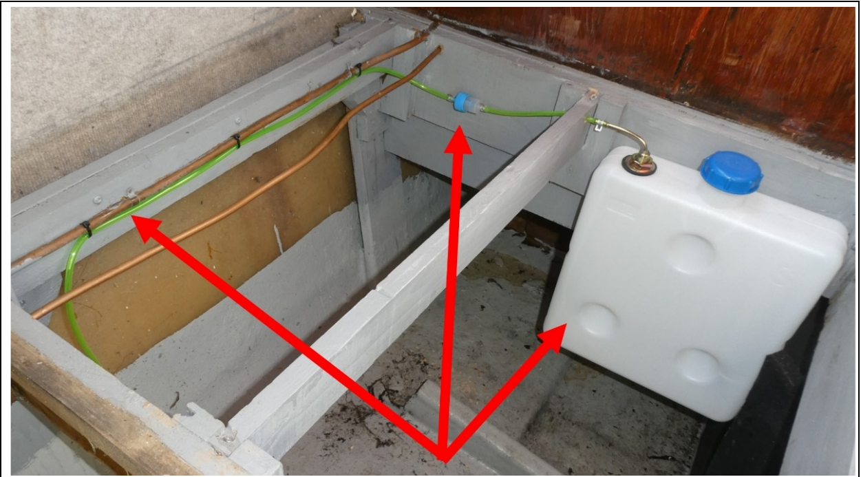
Fig 1. Example of a 10lt diesel heater tank which can be accepted as being of suitable proprietary manufacture. The tank is connected to a plastic fuel line incorporating a plastic filter all of which can be accepted as being of suitable proprietary manufacture as they are of a type known to be supplied by diesel heater manufactures. The plastic fuel line material and the filter are acceptable provided the tank does not have a capacity of more than 10lt.
