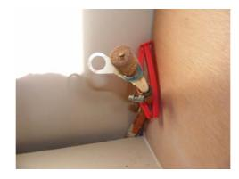
The photo shows an open-ended gas hose, blanked of by using a nozzle of a DIY sealant tube and a champagne cork.
